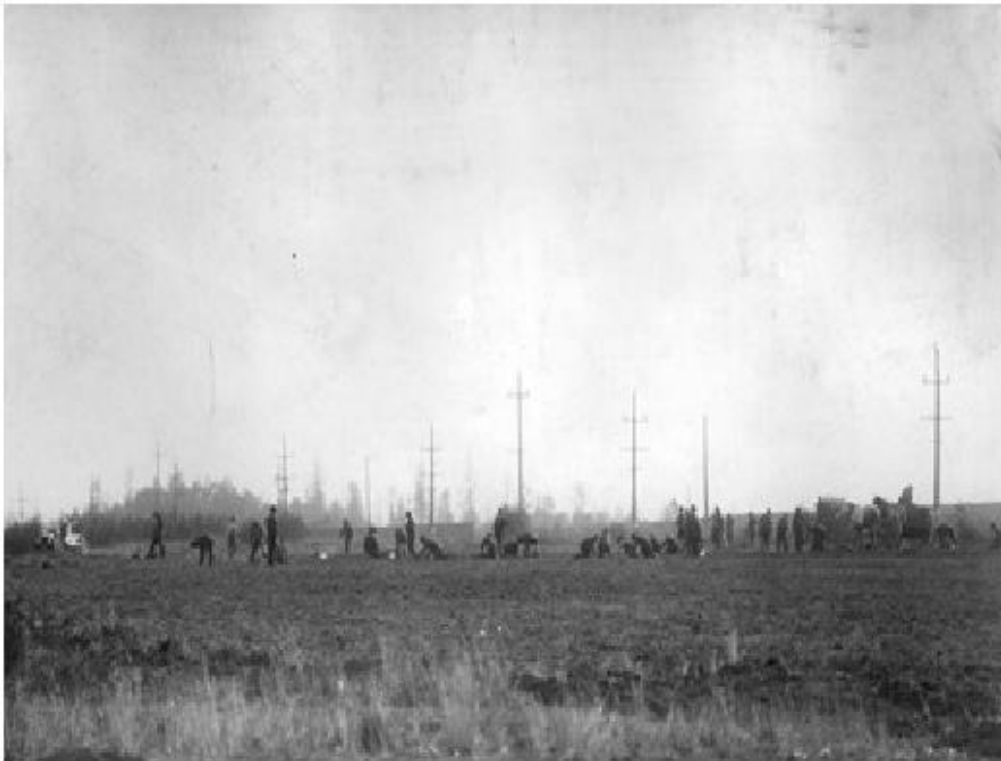
City prisoners working on Hole #1 in 1913 (photo courtesy of Seattle Municipal Archives)
